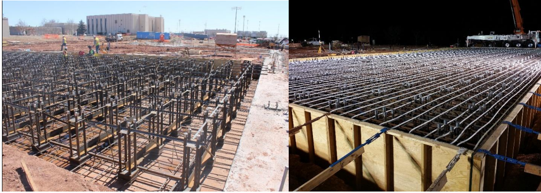
Fig. 1. Reinforcing detail in the mass floor.
